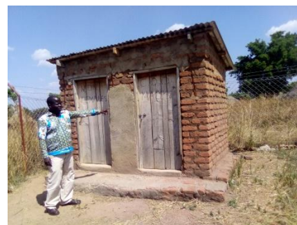
Figure 5: The old latrine at the Market shed still being used
