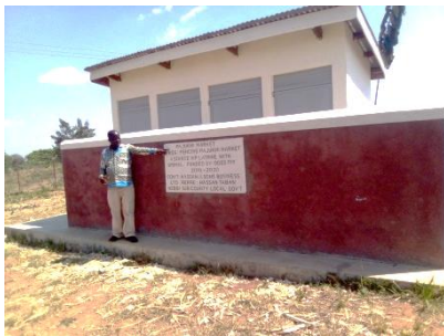
Figure 8: The new latrine to be used after community sensitisation
