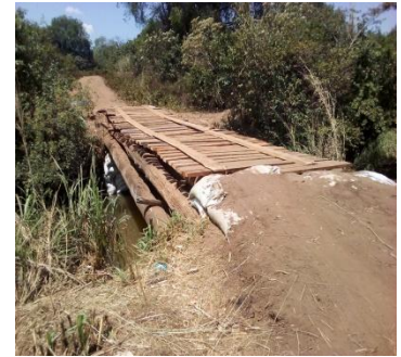
Figure 4: The repaired BRIDGE!
