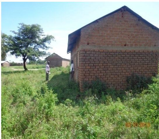
one block of staff house constructed by parents in Panyimur p/s
