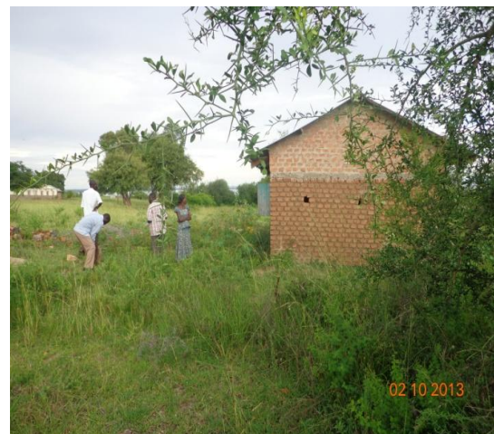
one block of staff house constructed by parents in Nyakagei p/s
