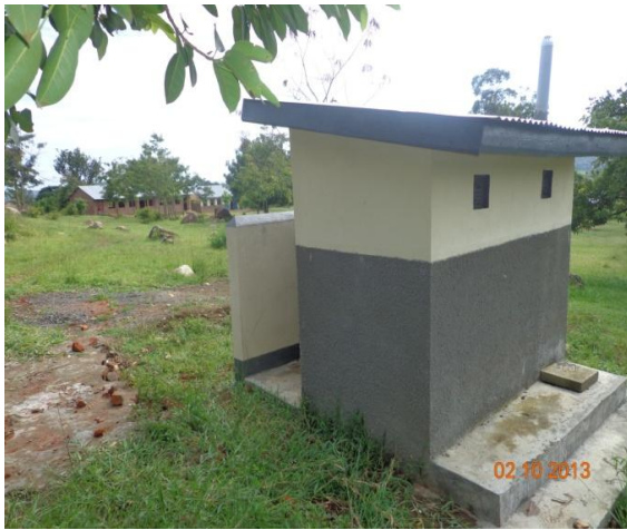
Completed two stances latrine under SFG for girls in Oweko p/s
