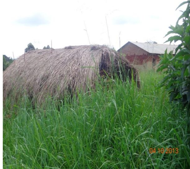
Temporary 2stances latrine for girls in Lwala p/s constructed by parents
