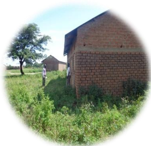
One block of staff house constructed by parents in Panyimur p/s one block of staff house constructed by parents in Nyakagei p/s
