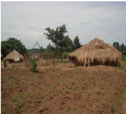
Teacher's house construction in Kango P/S
